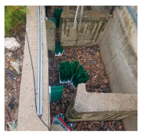
**Figure 3.** To restore the VSF of Cataloluk HPP, the brush blocks and substrate were placed in the pools. The bristle modulus of elasticity  $E_b = 1.45$  GPa (polypropylene), and the density of the bristle  $\rho_b = 905$  kg/m<sup>3</sup>. Arrow shows the flow direction.
