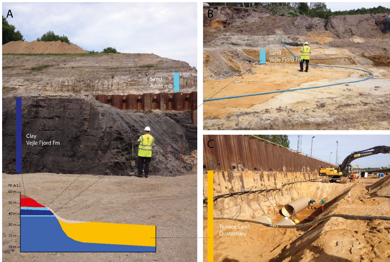
Figure 3. Post auditing the geological model on site. Sheet piling is visible in (A,C). Miocene sand from the Veile Fjord Fm (B) During construction, the groundwater table was lowered in several sections along the motorway with a suction cell system at the sheet piling, with suction cells every 1 m connected to larger pumps, picture (C).
