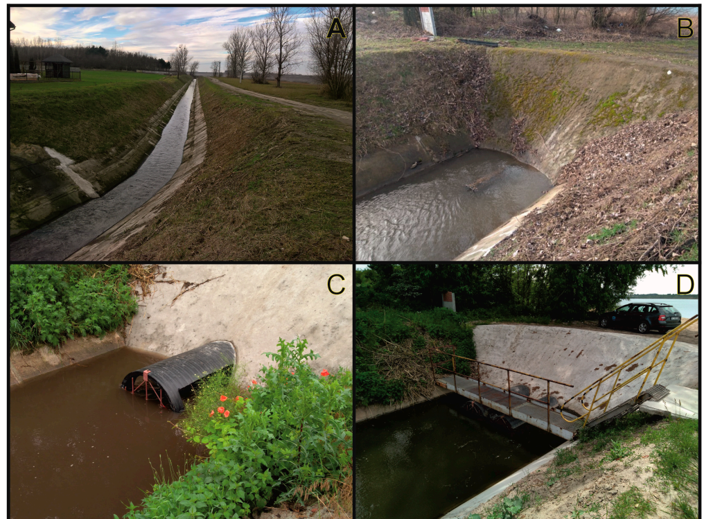
Figure 5. System supplying the post-mining reservoir Kleczew with mine waters from drainage of the opencast mine Józwin IIB: (A)—ditch supplying water, (B)—pipe supplying water in the period VII.2016–VI.2020 ( \Phi = 500 mm), (C)—pipe supplying water in the period VI.2020–XII.2020 ( \Phi = 1000 mm), (D)—pipes supplying water since XII.2020 ( 2 \times \Phi = 1000 mm).
