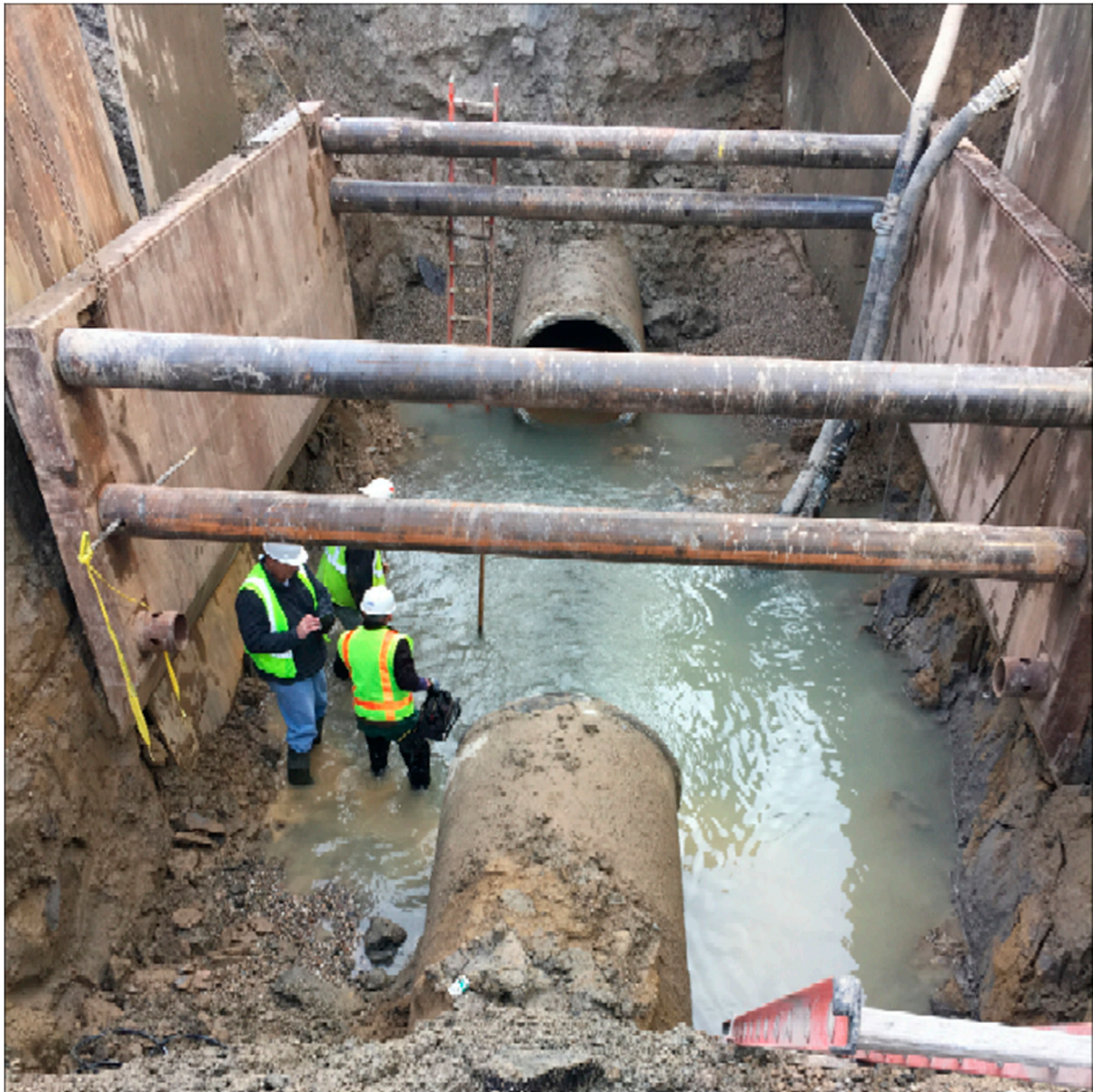
Figure 3. Excavation for Repairing Failed 1.2 m (48-inch) Water Pipeline (Photo Courtesy of GLWA).
