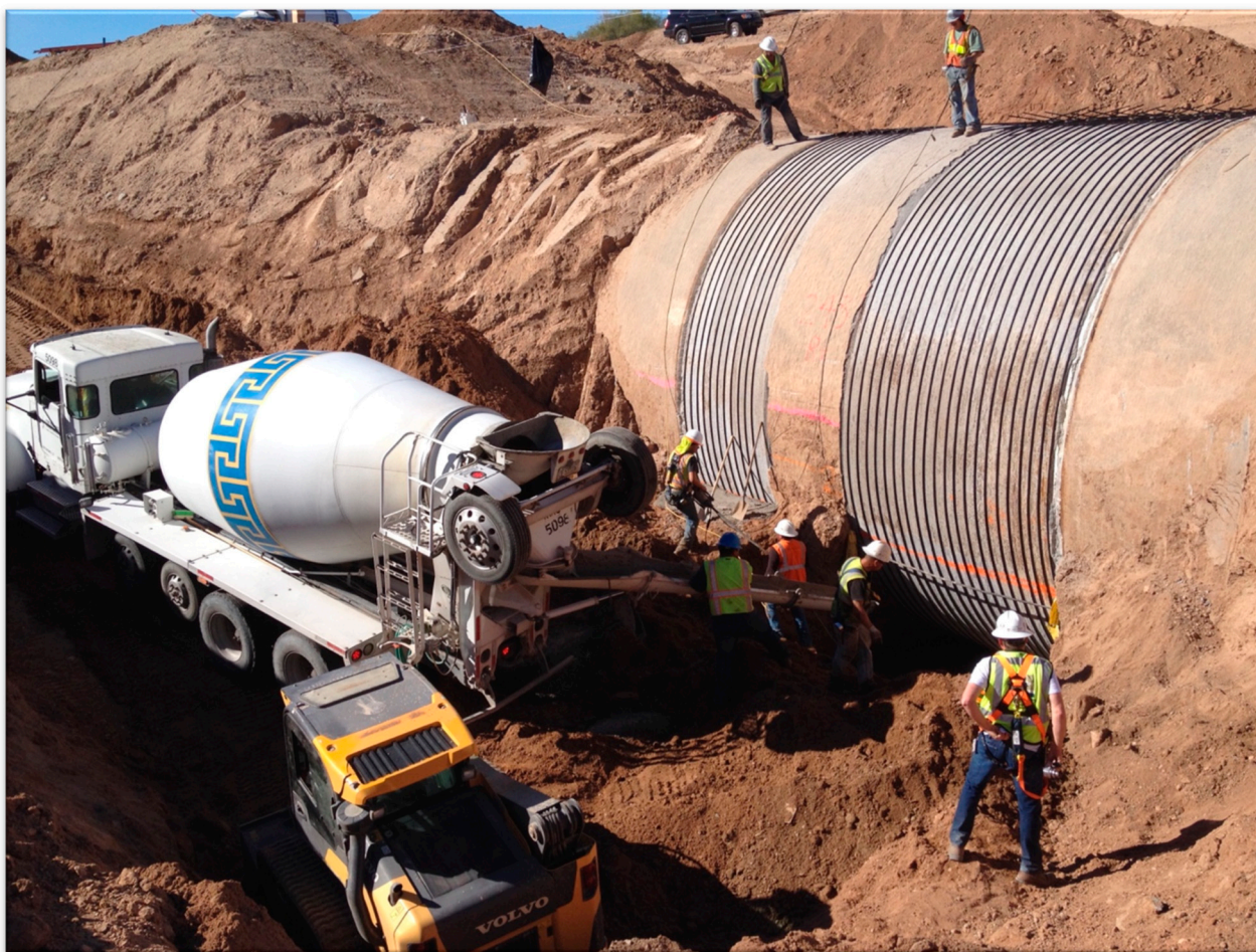
Figure 4. Planned Maintenance Activities on a 6.4 m (252 inch) Prestressed Concrete Pipe (Photo by J. Geisbush).
