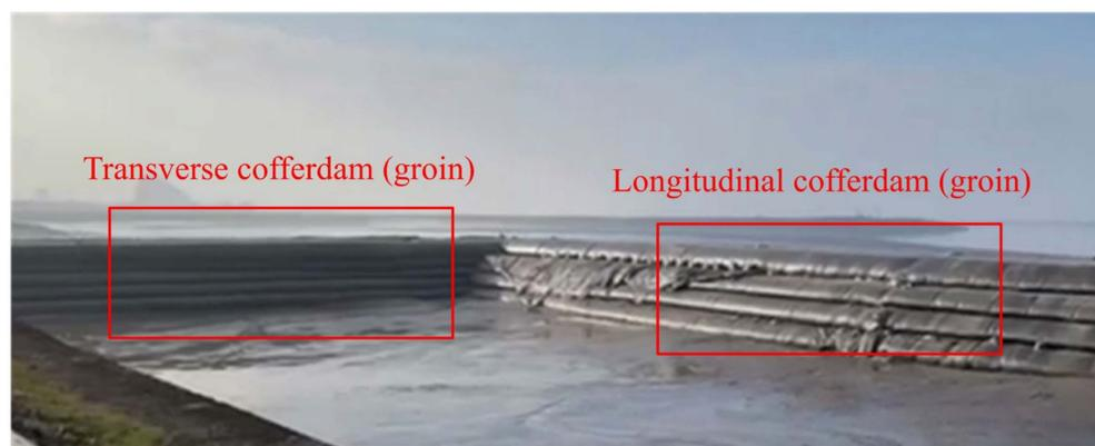
**Figure 1.** Transverse cofferdam and longitudinal cofferdam.
