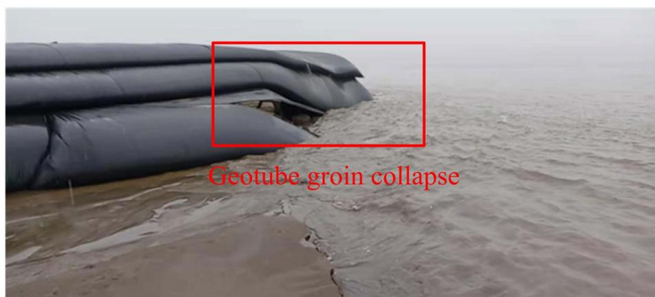
**Figure 2.** Geotube groin collapse.
