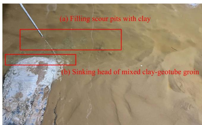
**Figure 20.** Scour pit at the head of the mixed clay–geotube groin.
