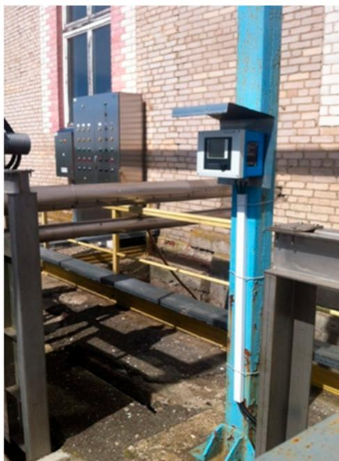
**Figure 8.** Measuring complexes of pH, ORP, conductivity, and temperature.
