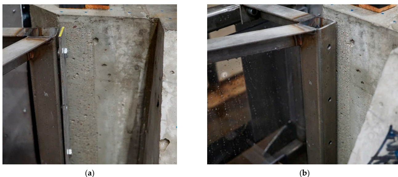
Figure 5. The right-hand side support (a) with the extension and (b) without the extension but with a roughened concrete surface.
