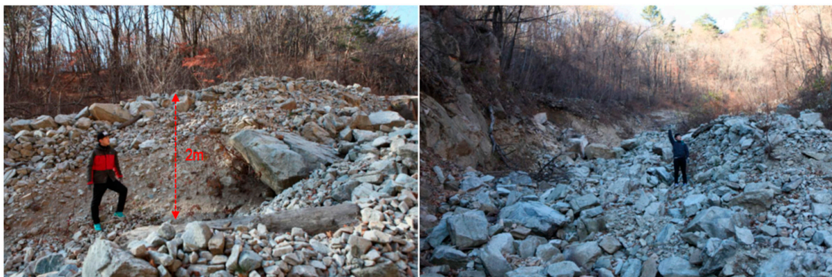
Figure 2. Photographs of debris flow-induced damage (erosion and sediment section).
