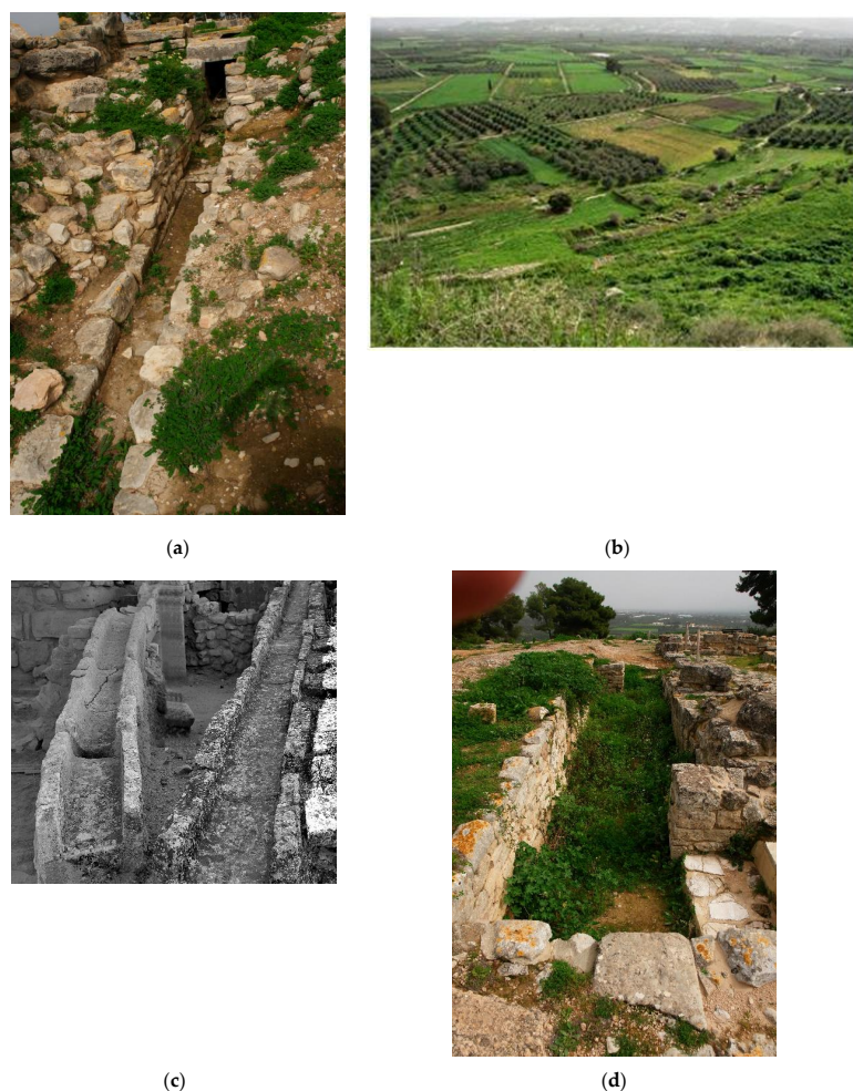
Figure 2. Water reuse in prehistoric times: (a) drainage channels in the palace of Phaistos and (b) downhill farmland irrigated by the flow; (c) drainage channels in Hagia Triada and (d) cistern in Hagia Triada for storage of water targeted for land application (Photos are of Andreas N. Angelakis).
