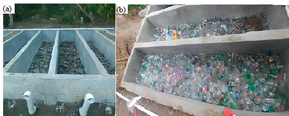
Figure 3. Filter media used in CWs: (a) PRR; (b) rough recycled PET waste.
