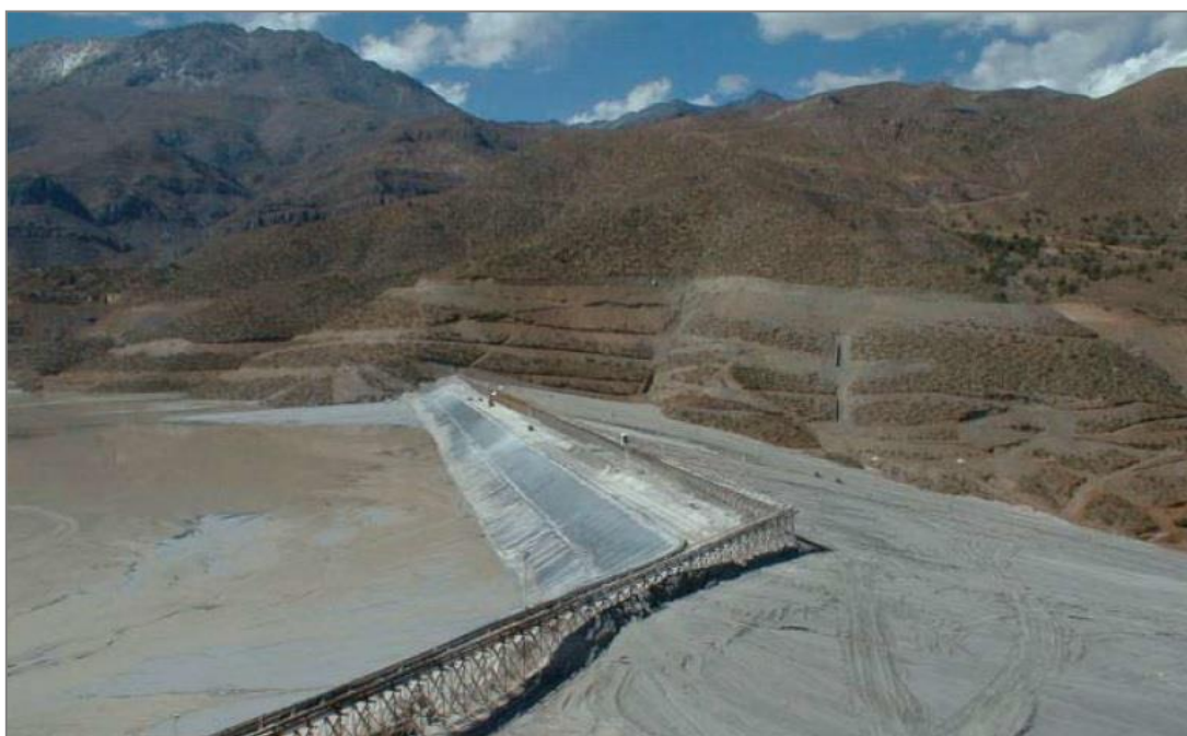
Figure 6. Copper mine tailings management—partially lined TSF—Los Quillayes TSF, Chile.
