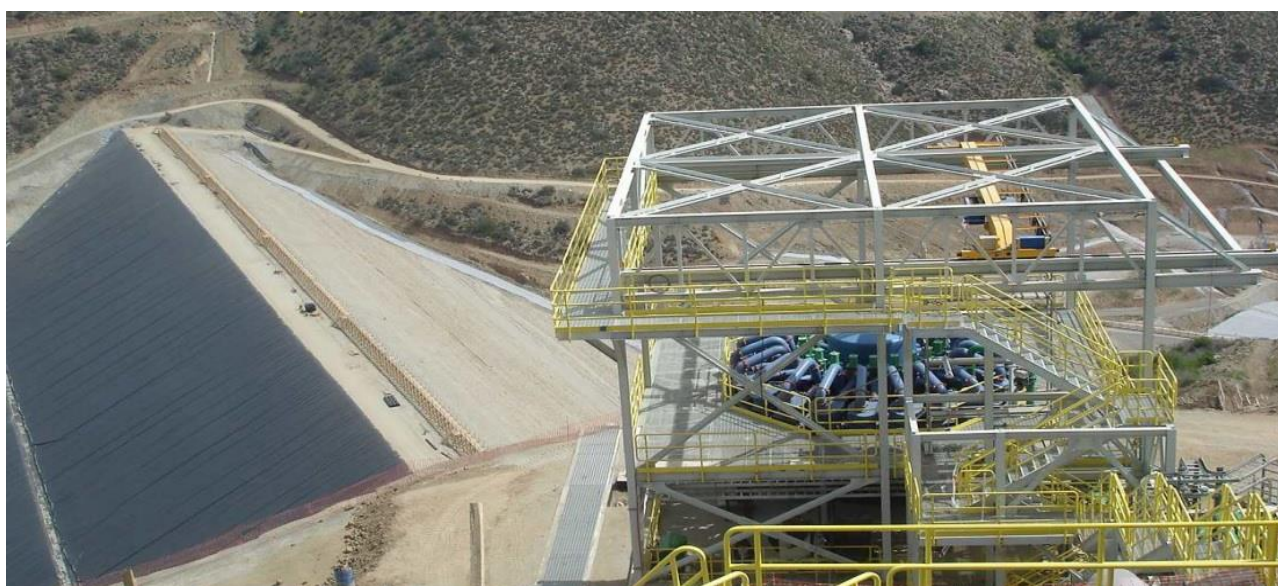
Figure 19. Panoramic view of TSF starter dam with geomembrane liner and mine tailings hydro-cyclone station—TSF, Chile.
