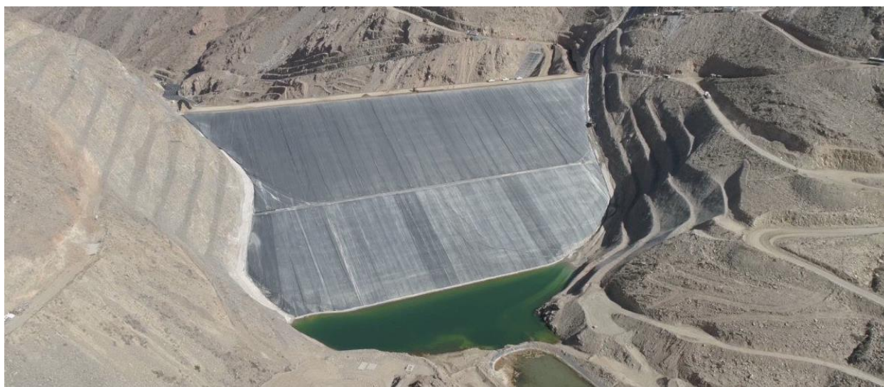
Figure 24. Front view—mine waste rock dam upstream face waterproofing construction detail—TSF, Peru.
