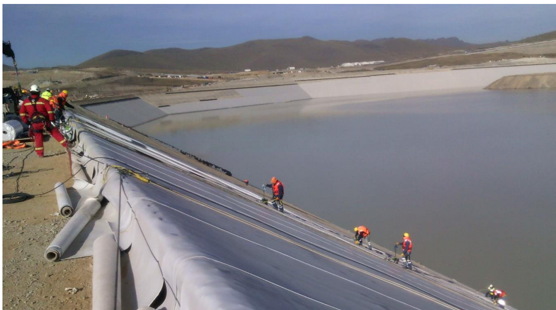
Figure 13. Geomembrane installation—typical construction activities, 2H:1V dam slope—Peru.
