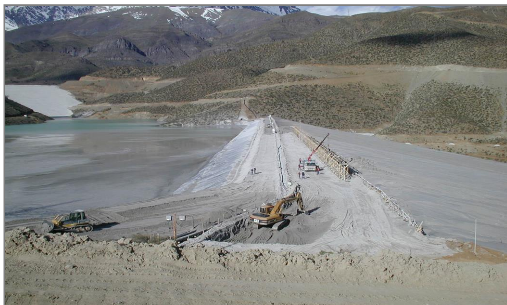
Figure 22. Cycloned tailings sand dam upstream face waterproofing construction process—TSF, Chile.
