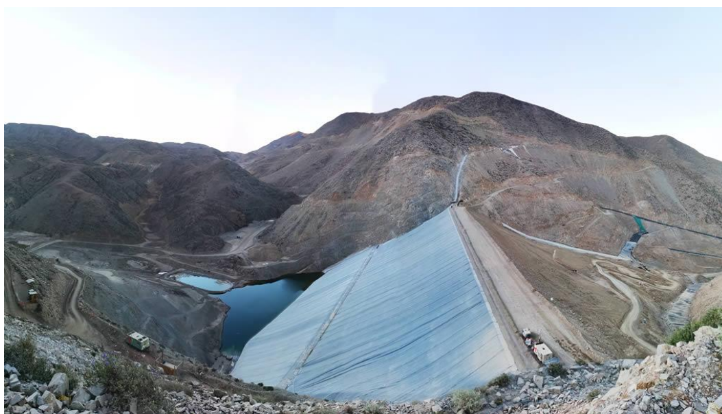
Figure 23. Panoramic view—mine waste rock dam upstream face waterproofing construction detail—TSF, Peru.
