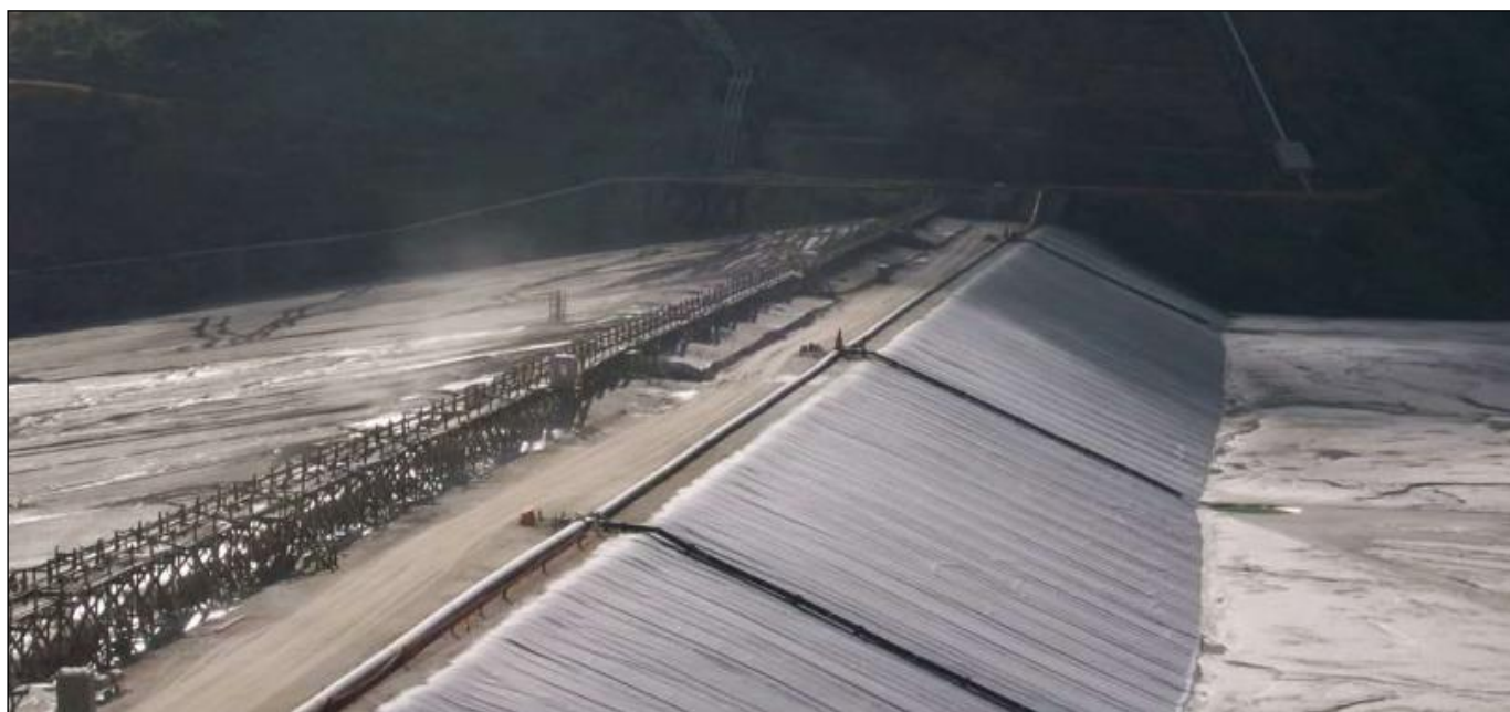
Figure 20. Cycloned tailings sand dam upstream face waterproofing—TSF, Chile [44].
