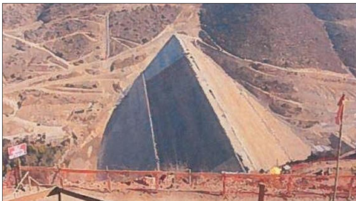
Figure 17. Starter dam upstream face geotextile–geomembrane liner installation second stage finished—TSF Starter Dam, Chile [42,43].
