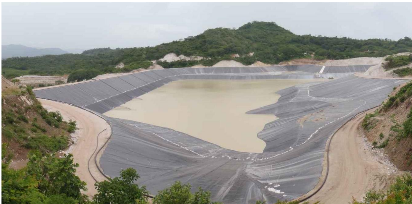
Figure 29. Example of use of geosynthetic liner in the zone of a TSF in contact with rock—TSF Peru.
