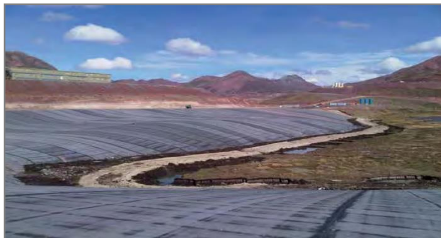
Figure 26. Mine waste rock dam upstream face waterproofing with bituminous geomembrane—TSF, Peru.
