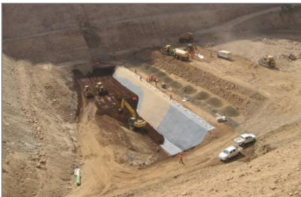
Figure 7. Example of cutoff trench and grout curtain system construction in a TSF.
