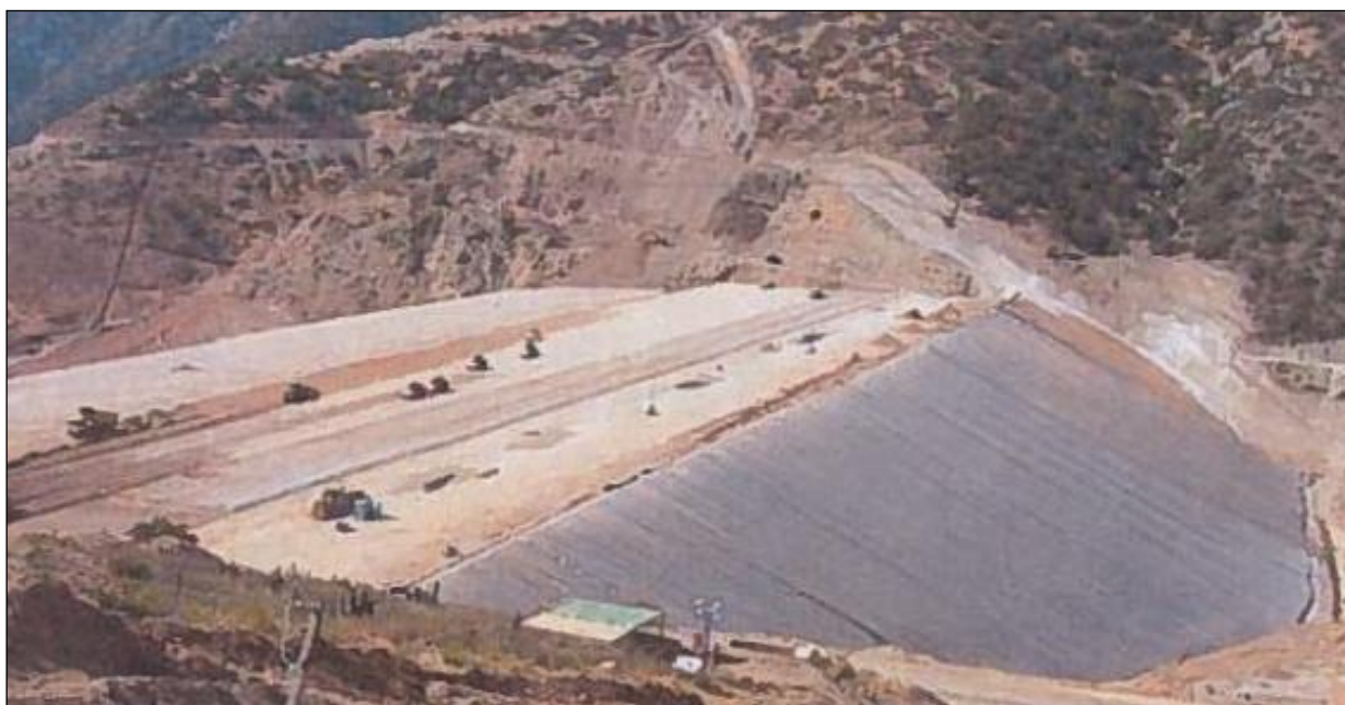
Figure 16. Starter dam upstream face geotextile–geomembrane liner installation first stage finished—TSF Starter Dam, Chile [42,43].
