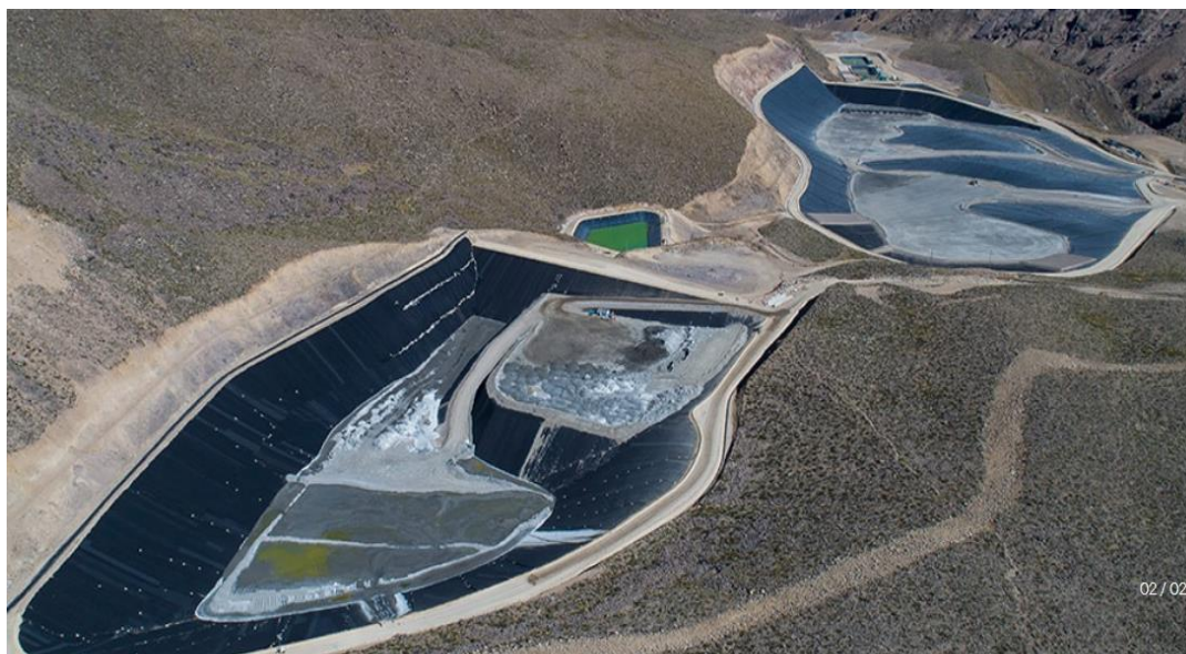
Figure 4. Gold mine tailings management—fully lined TSF—Tambomayo TSF, Peru [7].
