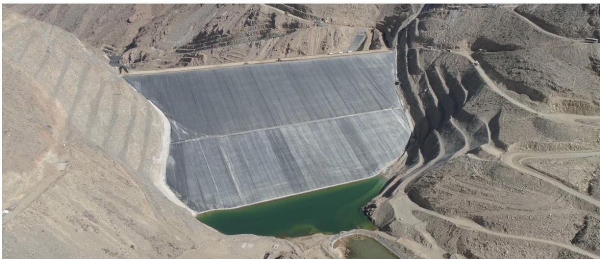
**Figure 24.** Front view—mine waste rock dam upstream face waterproofing construction detail—TSE, Peru.
