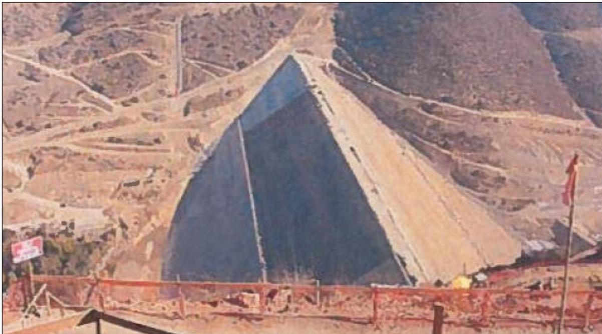
**Figure 17.** Starter dam upstream face geotextile–geomembrane liner installation second stage finished—TSF Starter Dam, Chile [42,43].
