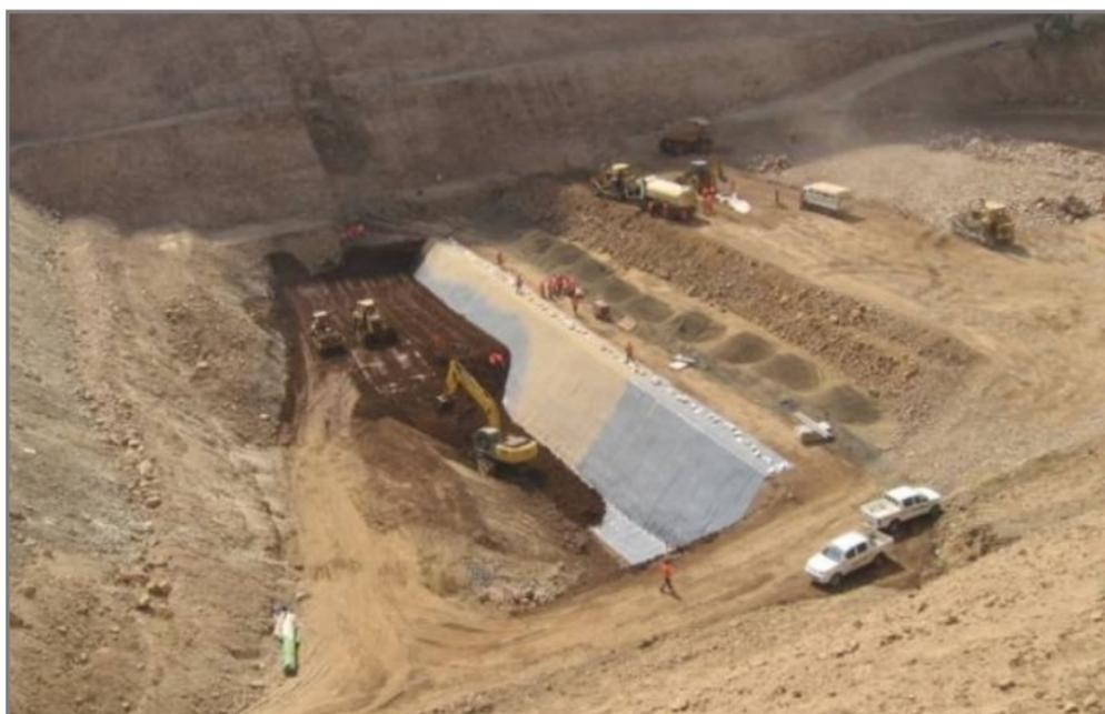
**Figure 7.** Example of cutoff trench and grout curtain system construction in a TSF.
