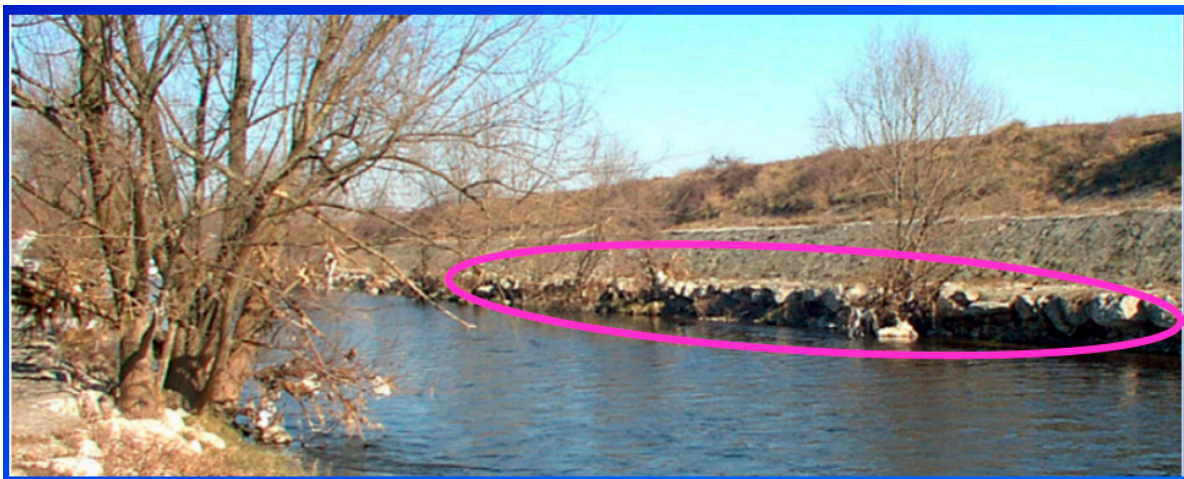
Figure 4. An example of consumption of the “work-in-good-shape” capital, because of lack of maintenance and periodic replacement (river Chiese, Italy): the toe of the bank protection is disrupted (fuchsia circle) and the door of a defense collapse is ajar.
