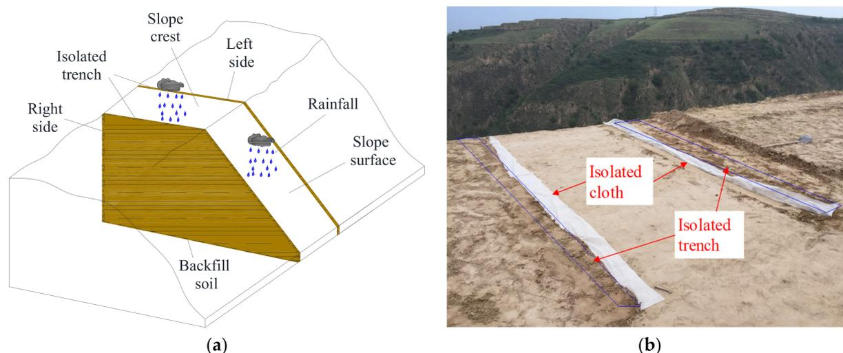
**Figure 1.** Treatment measure of deep-buried isolated trench. (a) Schematic diagram of the isolated trench; (b) the slope crest after construction with isolated trench.
