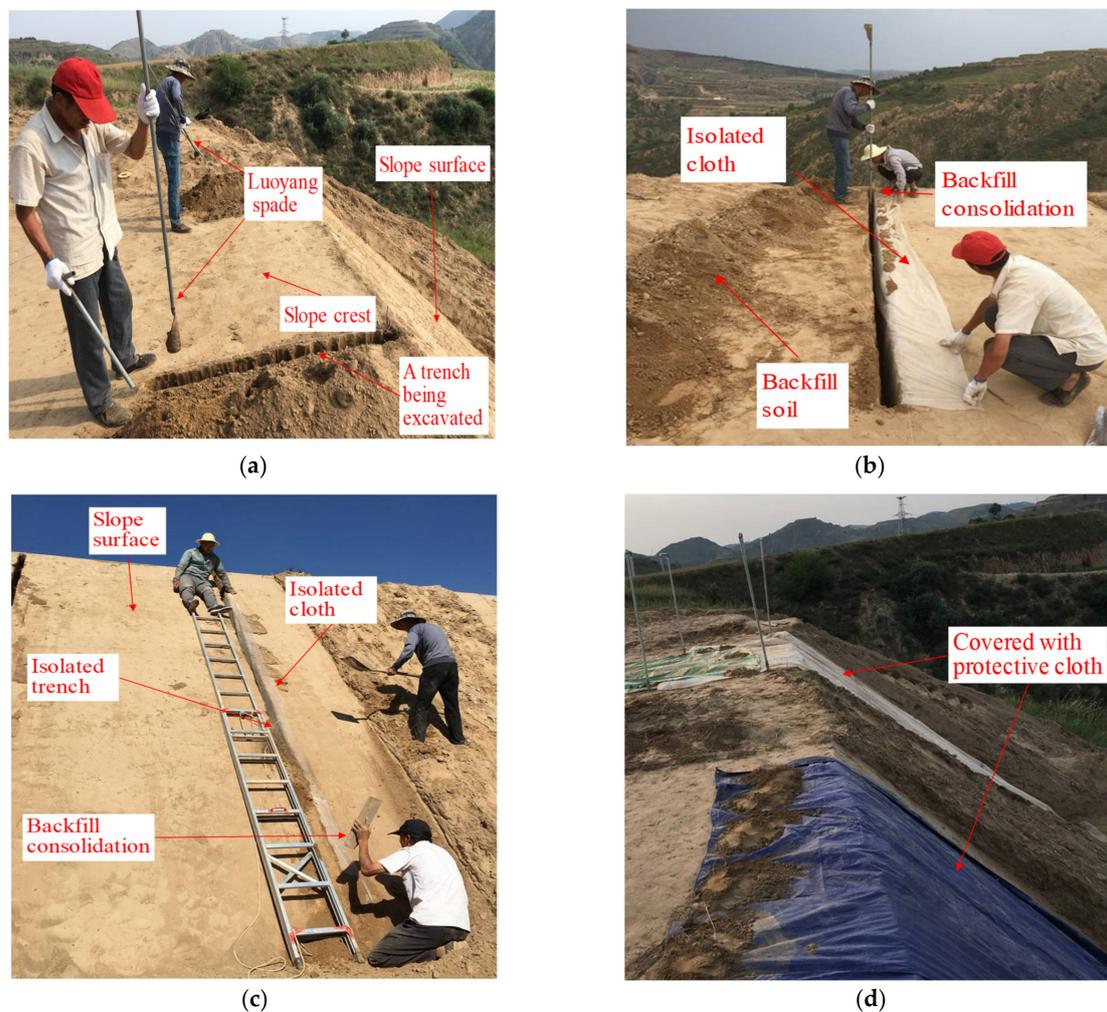
**Figure 3.** Construction process of isolated trench: (a) excavation of isolated trench; (b) laying isolated cloth and backfill soil at the slope crest; (c) laying isolated cloth and backfill soil at the slope surface; (d) protection after construction.
