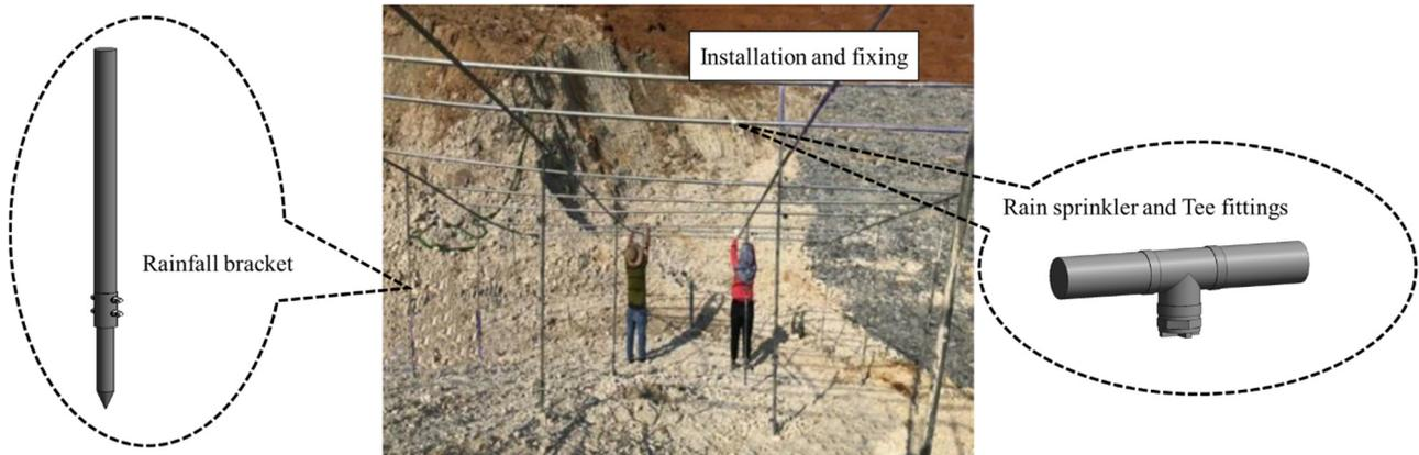
**Figure 6.** Site installation of the rainfall system.
