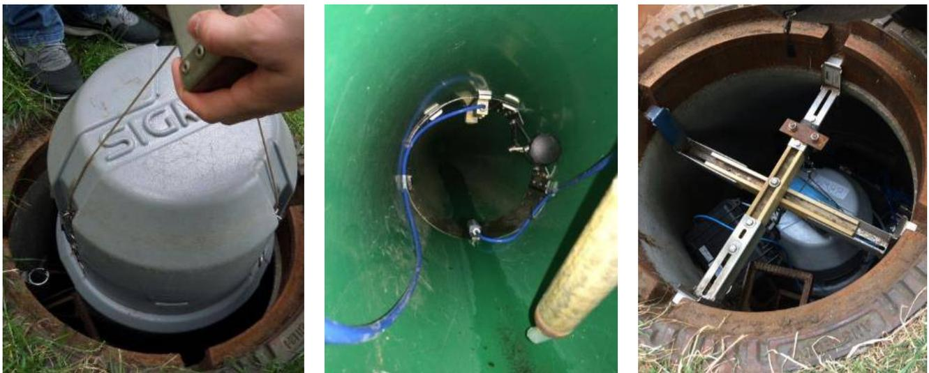
**Figure A4.** Installation of an automatic sampler and flow measuring device in a storm sewer and a manhole.
