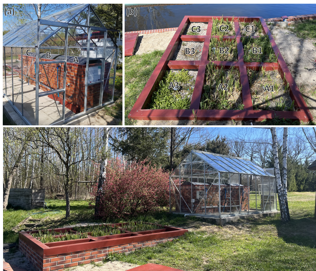
Figure 2. The NTSW pilot plant (adapted from Halicki and Halicki [12]). The three parallel wastewater treatment and water renewal processes are conducted in different daily hydraulic loads, namely 70, 100 and 130 L/m 2 for the A, B and C letters, respectively. (a) Compost beds. (b) Water renewal beds: denitrification beds (1), phosphorus beds (2) and activated carbon beds (3). (c) Setting of the NTSW pilot plant.
