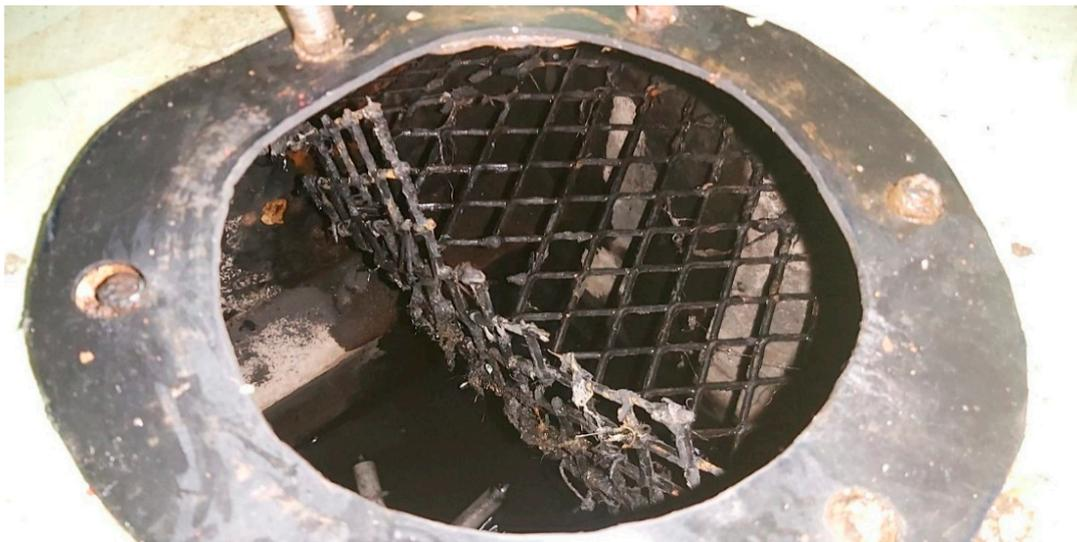
**Figure 9.** The coarse screen of mechanical purification plant.
