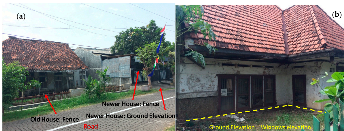
Figure 1. (a) An old house in a housing area that has been impacted by land subsidence, thus resulting in the ground elevation of the houses is lower than the road elevation, (b) the current condition of an older house whose window elevation is the same as the ground elevation due to land subsidence.
