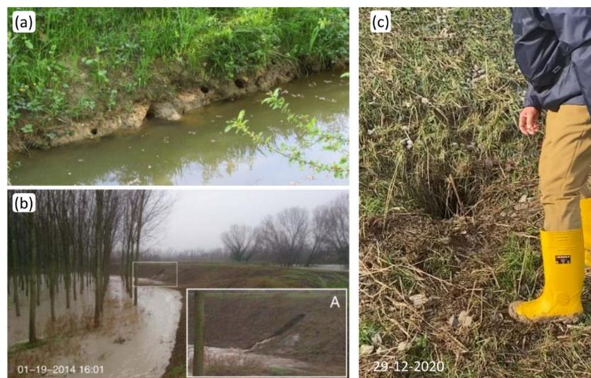
**Figure 2.** (a) Typical burrows produced by crayfish *Procambarus clarkii* on irrigation ditches (adapted from [4]); (b) concentrated erosion through a mammal burrow in Panaro levee near Modena (Italy) (adapted from [5]. WILEY 2005); (c) mammal burrow found on the land side of the Panaro levee near Modena (Italy).
