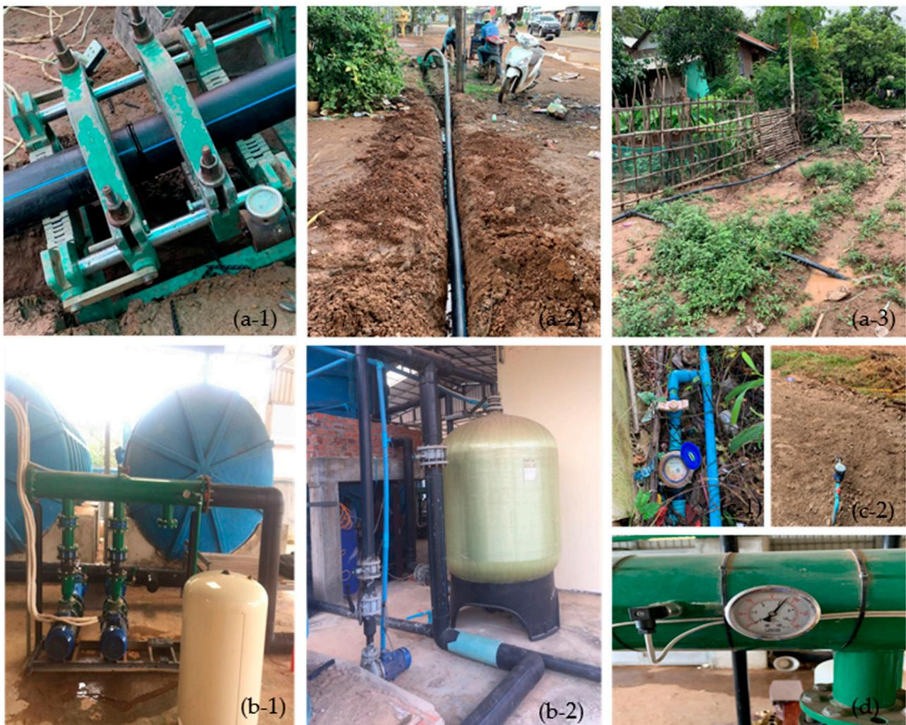
Figure A3. (a-1 to a-3) Distribution pipe installation; (b-1 and b-2) water purification installation; (c-1 and c-2) water meter installation; and (d) water pressure meter.
