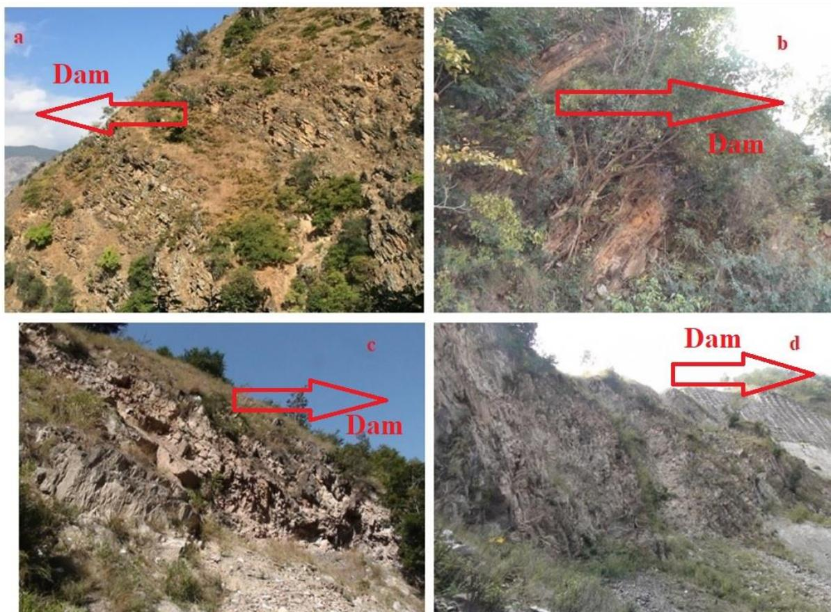
**Figure 3.** (a) The toppling deformation body of the upstream side of the Keli River on the left bank. (b) The toppling deformation body of the downstream side of the second gully at the dam on the left bank. (c) The toppling deformation body of the upstream side of the Tiemenka River on the right bank. (d) The toppling deformation body of the downstream side of the Tiemenka River on the right bank.
