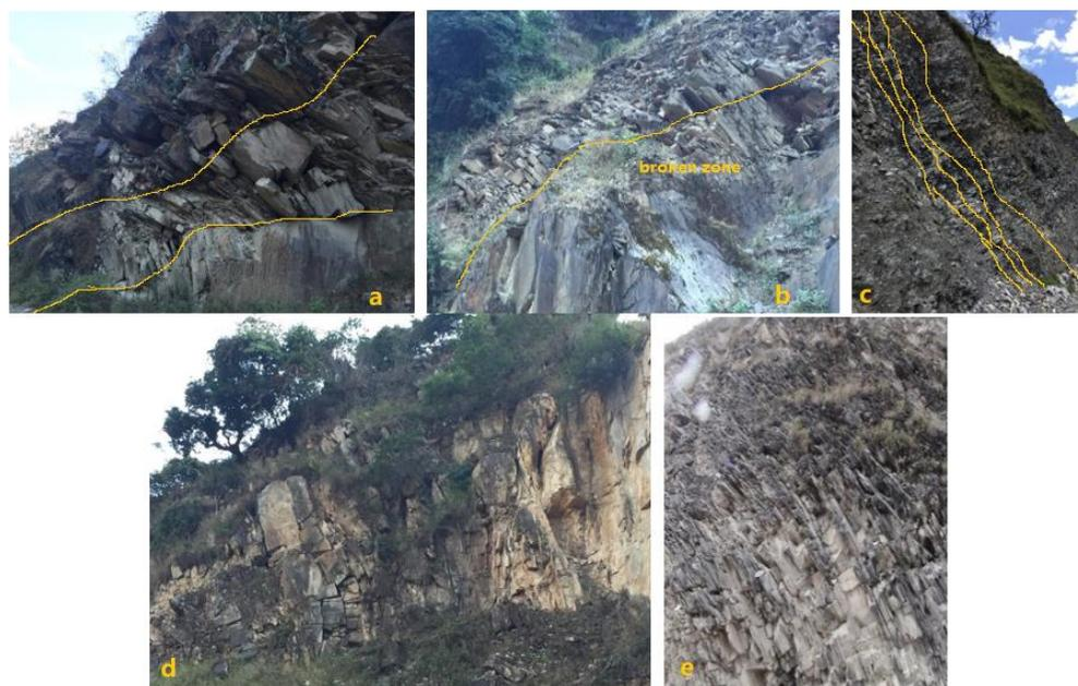
**Figure 5.** (a) The angle of the toppling fracture surface is less than  $10^\circ$  in the reverse slope. (b) The change trend of the dip angle of the rock layer. (c) The dip angle of the toppling broken failure surface is  $63^\circ$  above the altitude of 1430 m. (d) The toppling-loose rock mass of the old highway slope on the downstream side of the Wanba River. (e) The toppling-relaxation rock mass of QD5-1 in the transversal.
