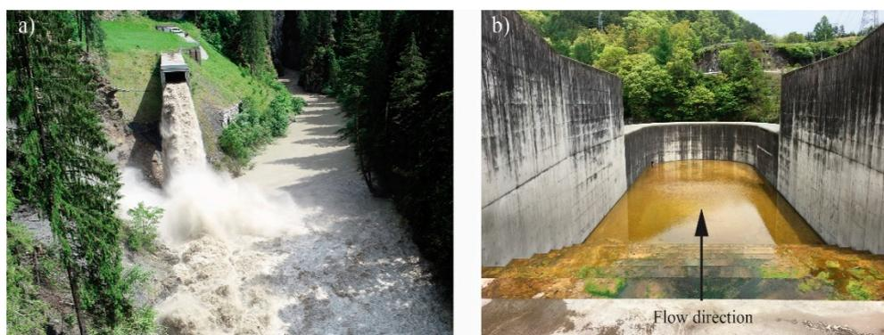
**Figure 3.** Outlet structures of (a) Solis SBT in Switzerland and (b) Miwa SBT in Japan.
