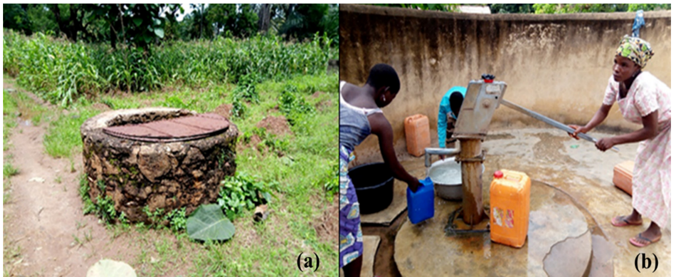
Figure 4. Traditional sinks exploiting the water of the alterite reservoir at Niamtougou (northwest of the study zone) (a) and borehole equipped with a human-operated pump, exploiting the water of the fractured reservoir at Bébédá (center of the study zone) (b).
