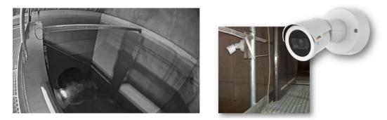
Figure 11. IR camera with an image of the forebay tank emptied.
