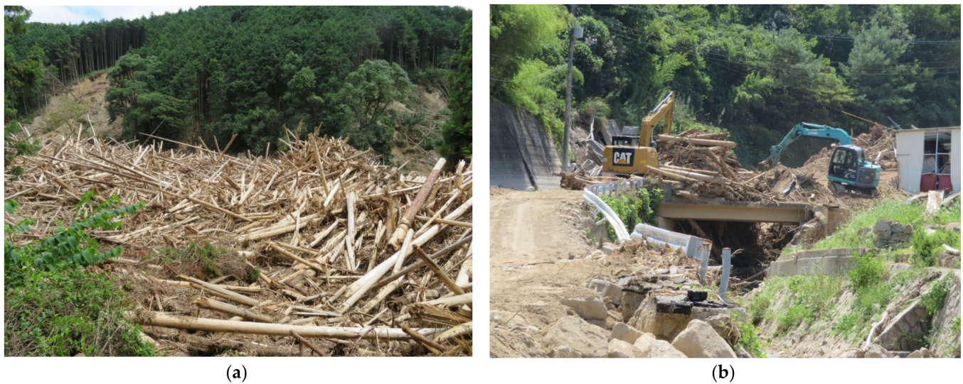
Figure 1. (a) A large amount of LW that accumulated in Asakura City (Fukuoka Prefecture) during heavy rainfall in northern Kyushu in 2017; (b) LW blocking the bridge over a small river during heavy rain in Hiroshima Prefecture in 2018 (The photo shows the blocking LW being removed).
