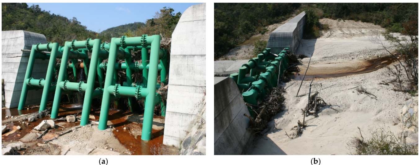
Figure 2. (a) LW captured by an open sabo dam (check dam) during heavy rainfall in Hofu City (Yamaguchi Prefecture) in 2009; (b) A large amount of sediment accumulated with the driftwood, completely clogging the check dam.
