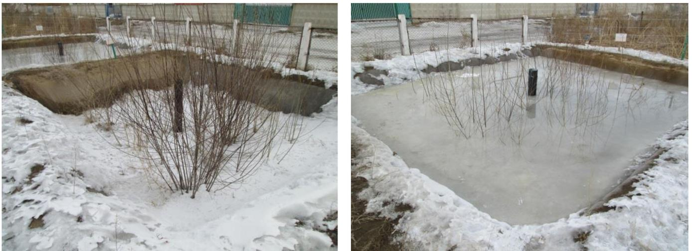
Figure 4. The pilot treatment beds. Bed A operated with external winter storage and summer irrigation (left) and bed B operated with internal winter storage, where the wastewater is stored on top of the treatment area during winter.
