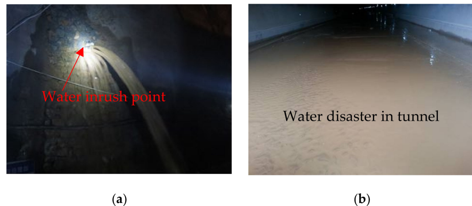
Figure 3. Site condition of water inrush in the Shangjiawan tunnel (a) water inrush point; (b) water disaster in tunnel.
