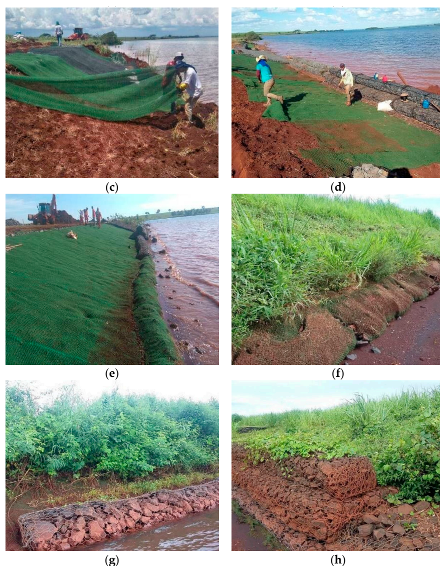
Figure A1. General installation procedures of the techniques: (a) mechanical reshaping of the margins, (b) construction of the anchor trench, (c) margin anchorage of the geomat, (d) sack gaban installation under the geomat, (e) final installation of the geomat erosion control technique, (f) geomat erosion control technique after two years of installation, (g) geomat and sack gaban after two years of installation, and (h) geomat and sack gaban after four years of installation.
