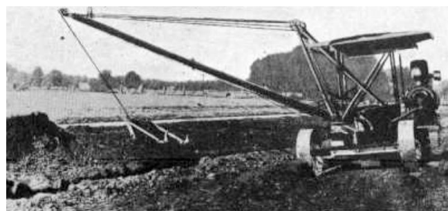
Figure 12. Power-operated backfiller filling a large tile ditch [65].
