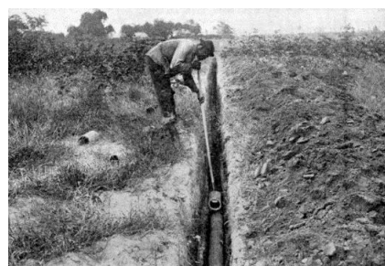
Figure 8. Laborer laying tile [64].
