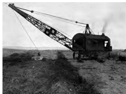
Figure 11. Filling up closed drain with dragline excavator [56].
