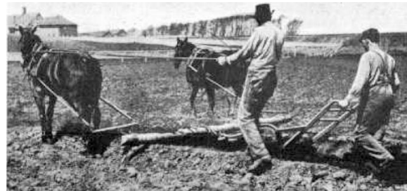
Figure 9. Filling up the ditch with a plow [19].
