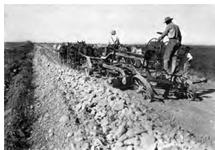
Figure 10. Filling up closed drain with teams and road grader [56].
