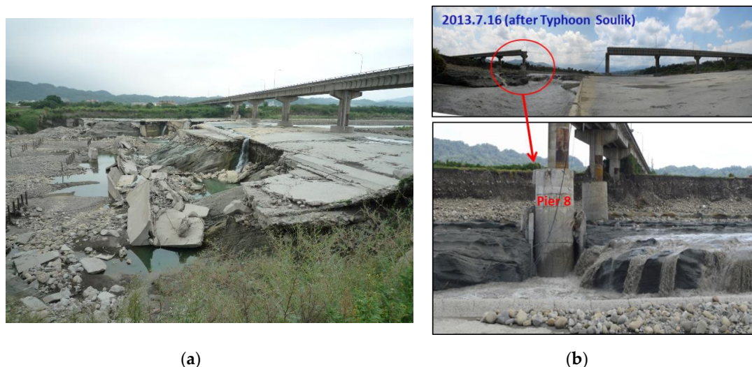
Figure 2. Scour downstream of grade-control structure leading to failure of Zhongzheng Bridge in Touqian River, Taiwan (a) scour downstream of grade-control structure in 2009 (courtesy of Yee-Meng Chiew); (b) Scour leading to bridge failure in 2013 (courtesy of Dr. Hong JH).
