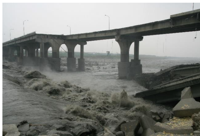
Figure 1. Failure of Houfeng Bridge in Dajia River, Taiwan due to pier-scour in September 2008 (courtesy of Yee-Meng Chiew).
