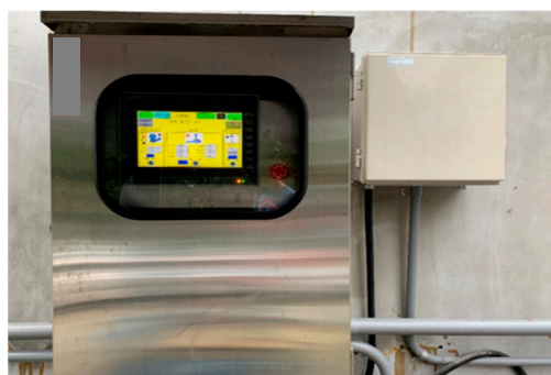
Figure 3. The human-machine interface (HMI) (yellow panel) of the programmable logic controller (PLC) for automatic SBR operation control.
