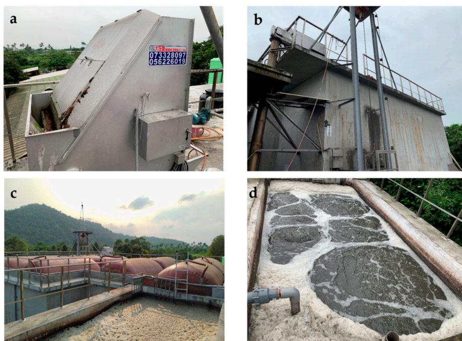
Figure 2. The appearance of the newly designed and constructed piggy wastewater treatment system. From left to right and up to down, they were solid/liquid separator (a), wastewater basins (b), anaerobic digesters (covered with brick-red plastic cover on the top of the digesters for collecting biogas) (c), primary clarifier (c), and sequencing batch reactor (SBR) (d).
