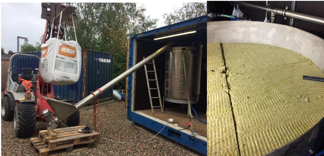
**Figure S2.** Filling of the sand biofilter (**left**) and the stonewool biofilter from the top (**right**).
