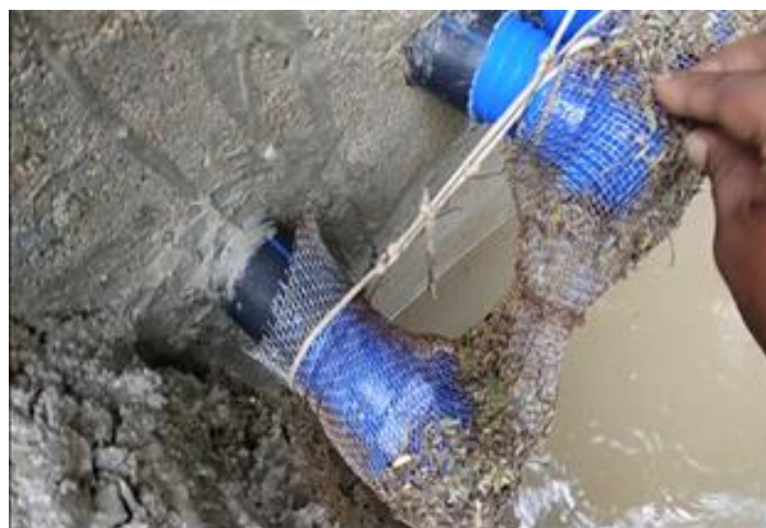
Figure 9. Recharge pit with filters. and clogging of the flow meter inlet.
