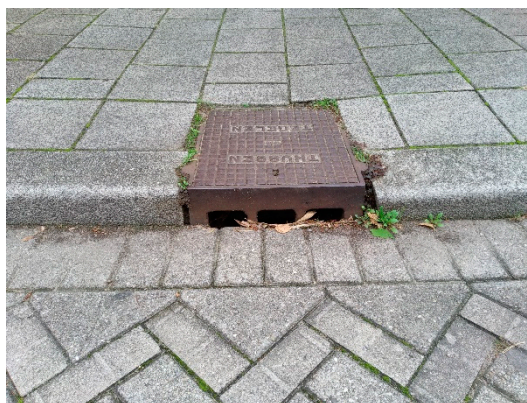
Figure 1. Roadside gully pot.
