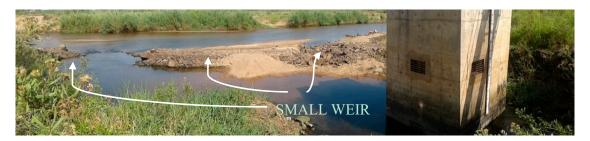
Figure 5. Picture of small weir next to the intake structure (Silva-Novoa. 24 January 2018).
