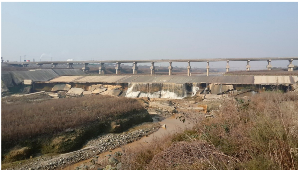
Figure 1. Scour at the grade control structure (GCS) downstream of the 105th Provincial Highway Bridge after the flood event on 9 July 2013 (discharge Q = 2710 \text{ m}^3/\text{s} ).
