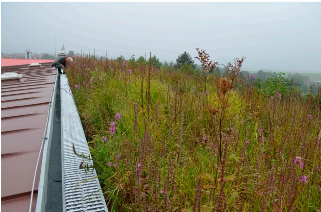
**Figure 4.** Building with half the roof area covered by a wetland roof (photo: Michael Blumberg).
