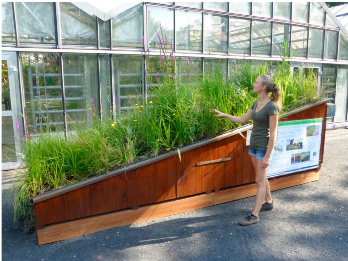
**Figure 5.** Pilot plant system of a wetland roof (planted area 4.5 m<sup>2</sup>) (photo: Andreas Zehnsdorf).
