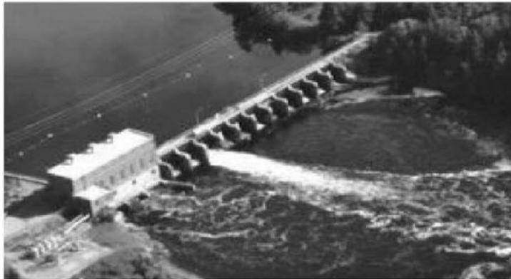
**Figure 2.** Practical sample of a hydraulic jump below abrupt asymmetric expansion [31]. Reprinted with permission from American Society of Civil Engineers (ASCE).
