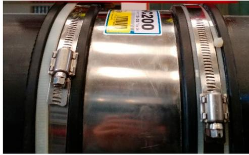
**Figure 2.** Flexseal Couplings SC200 reinforcement.
