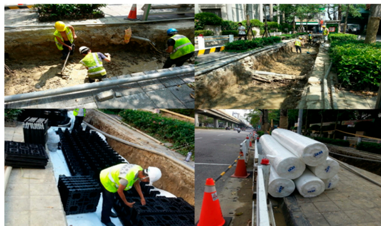
Figure 3. Installation of the underground stormwater storage tanks.
