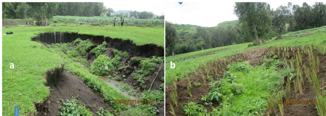
Figure 6. Gully RV2: (a) without treatment in July 2014 and (b) integrated gully head protection with regrading, stone riprap and vegetation in 2015.
