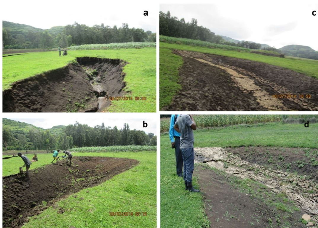
Figure 7. Gully RVB1 treated with head, bank and bed stabilization measures: (a) the original gully, (b) start of regrading the gully head and bank, (c) after the gully is treated in June 2014, and (d) in October 2014 the bamboo sheet covering the bed has broken down, but the head protection remained in place.
