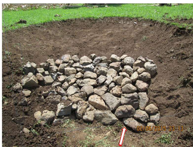
Figure 2. Initial stages of placing stones at the foot of the gully head to prevent any local gully bed and toe erosion.
