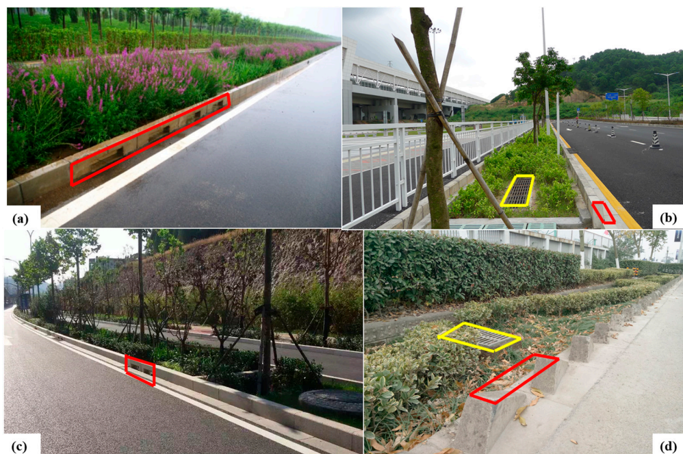
Figure 2. Continuous road-bioretention strip in (a) Beijing (curb inlet length L_{ci} = 0.5 m) taken by Yongwei Gong, (b) Shenzhen ( L_{ci} = 0.4 m) taken by Yongwei Gong, (c) Jinan ( L_{ci} = 0.4 m) taken by Xiaoning Li, and (d) Ningbo ( L_{ci} = 0.3 m) taken by Jianlong Wang. Red boxes show curb inlets and yellow boxes show overflow grate inlets in the bioretention cells.
