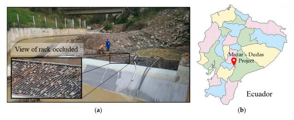
**Figure 2.** Mazar–Dudas Hydroelectric Project: (a) San Antonio bottom rack intake embedded in a weir—cleaning tasks and repairing process after a flood in the Mazar River, Ecuador (Image courtesy of Corporación Hidroeléctrica del Ecuador-CELEC EP Hidroazogues) [3]; (b) project location in Ecuador (without scale).
