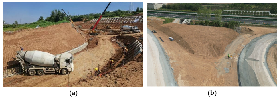
Figure 1. Actual open operation surface of the target highway construction site. (a) Panoramic view of the construction access road. (b) Local view of the open operation area.
