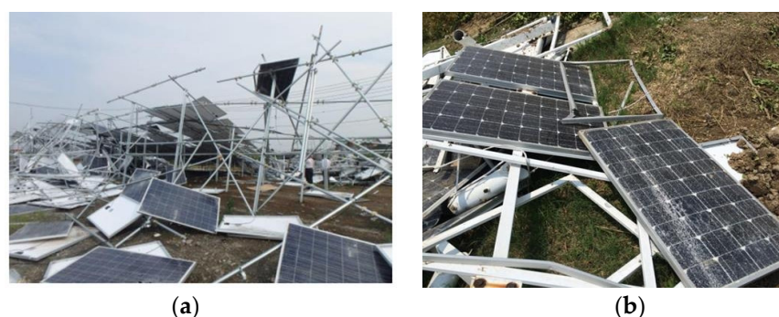
Figure 3. Example of wind-induced damages on PV panel arrays: (a) In Iseisaki city, Gunma prefecture, Japan in 2015; (b) In Yancheng city, Jiangsu province, China in 2015.
