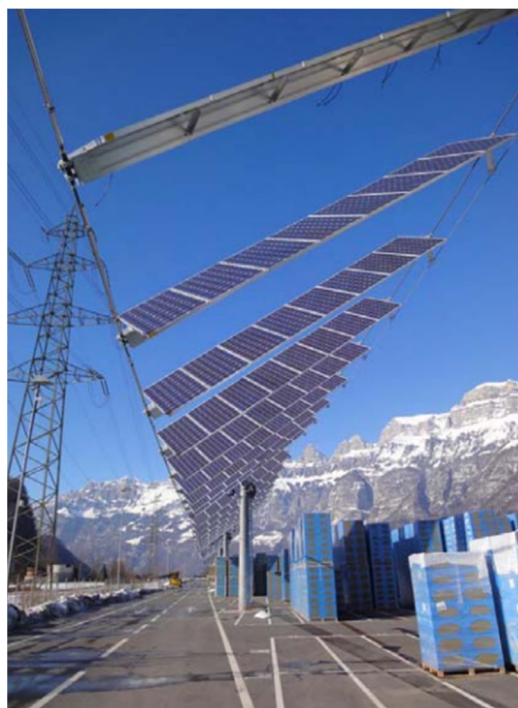
Figure 1. Example of the flexible PV system installation [7].
