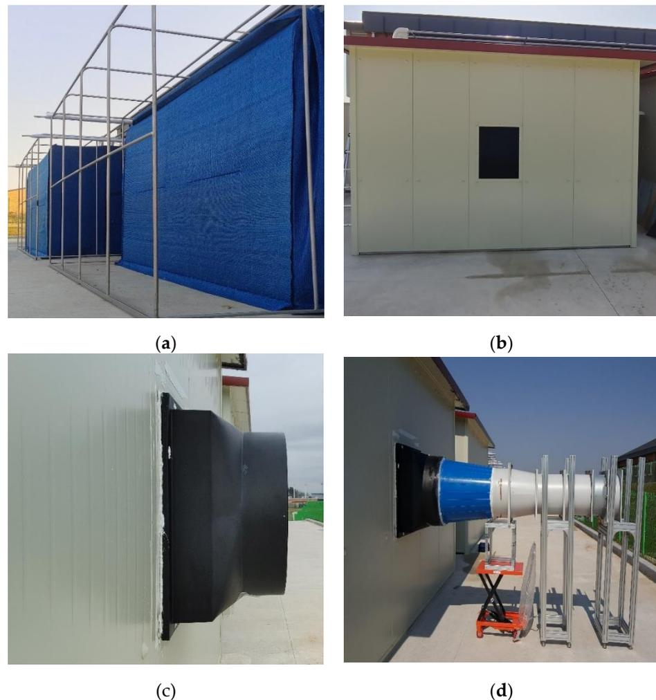
**Figure 2.** Curtain constructed on the outside of swine facility. (a) curtain, (b) metallic cover concealed the curtain, (c) single hole on the front of metallic cover, (d) ventilation measurement setup for air discharged through the single hole of metallic cover.
