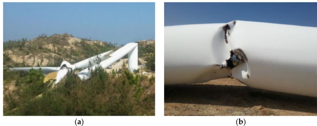
**Figure 4.** Photographs displaying tower damage due to Typhoon Usagi [23]: (a) tower collapse; (b) buckling failure.
