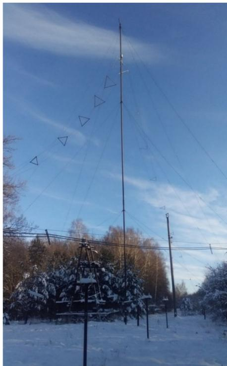
**Figure 3.** Antenna in village Vasilsursk: vertical Delta located on the 40-m mast.
