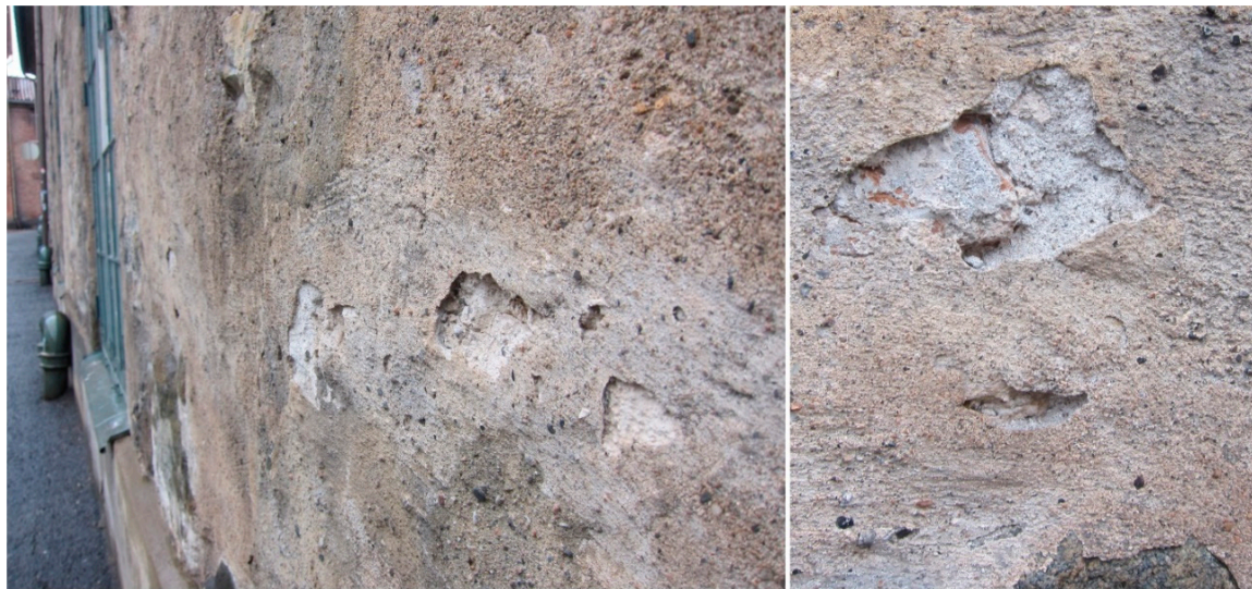
Figure 3. Initial and probably accelerating deterioration of a rough sand-containing rendering applied on the uneven surface of the building seen in Figure 4d, with protruding parts of stones from the wall under the rendering.
